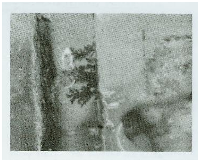
Figure 5. The dendritic appearance of corrosion products in the epoxy adhesive
