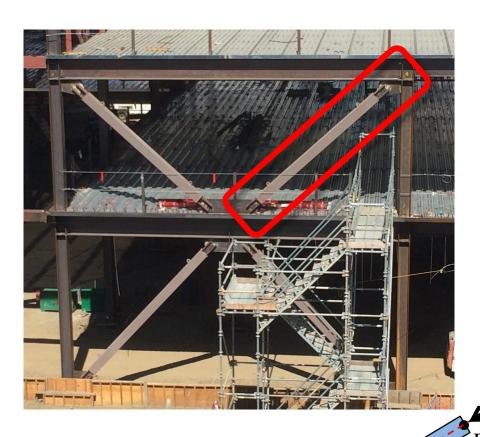
Braces in frames to resist seismic loads are often idealized as two-force members
