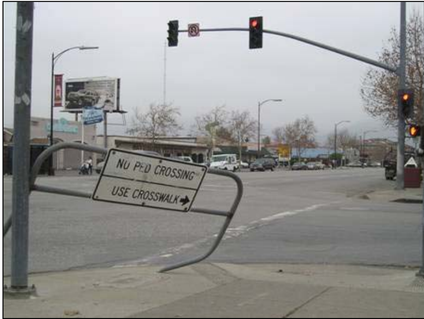
Figure 17: Intersection of Alum Rock Ave. and Sunset Ave. Pedestrians are forced to go out of their way to use a crosswalk to cross Alum Rock Ave. Crosswalk striping is deteriorated.
