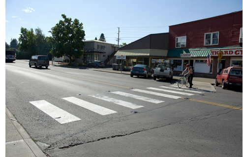
Pedestrian actuated in-pavement flashers alert motorists of a crossing pedestrian.
