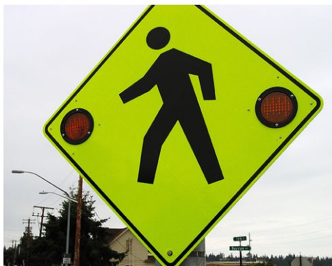
Pedestrian actuated flashing signs and beacons alert motorists of uncontrolled crosswalks,
