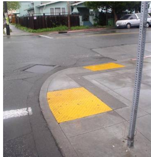
Truncated domes alert visually impaired pedestrians of an upcoming roadway.
