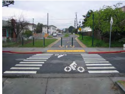
Berkeley's multi-use path crosswalk marking. West Street Path between University Avenue and Delaware Street
