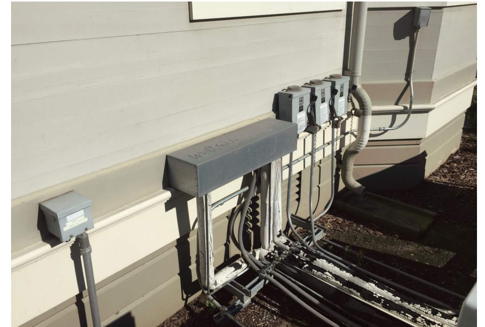
West facade utility ingress locations, 2017 (Page & Turnbull)
