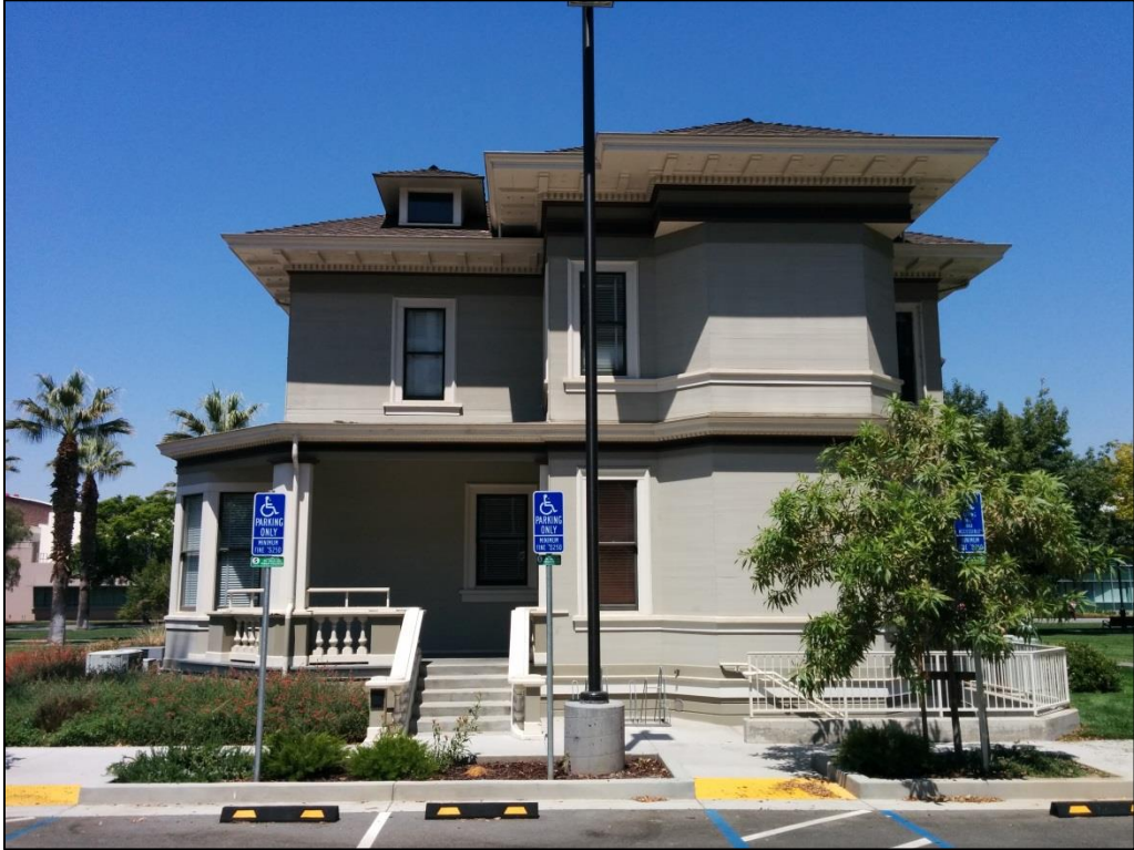
Figure 7. South elevation. View to the north.
