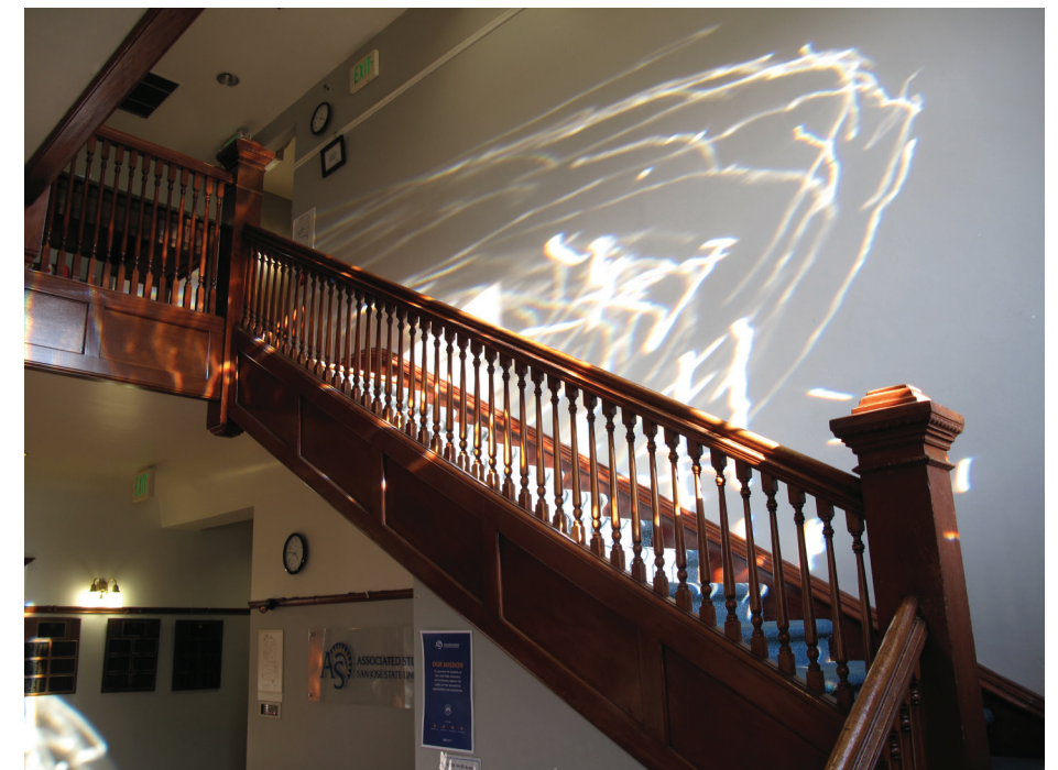
Front entry stairway and art glass window reflections, 2017 (Page & Turnbull)
