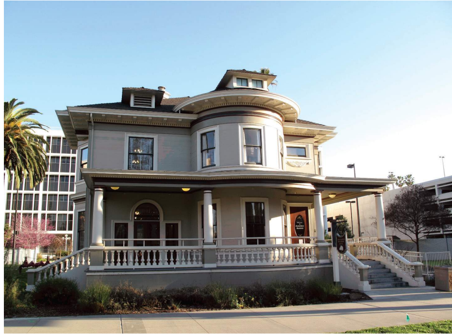
Primary (northwest) facade, looking southeast.
