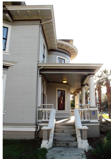
Front porch at northeastern corner, looking west.
