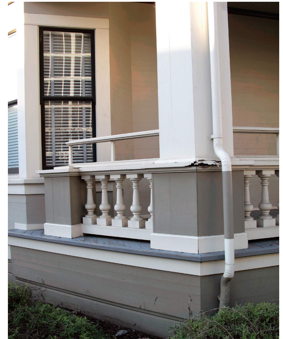
Rear porch, southwest corner, 2017 (Page & Turnbull)
