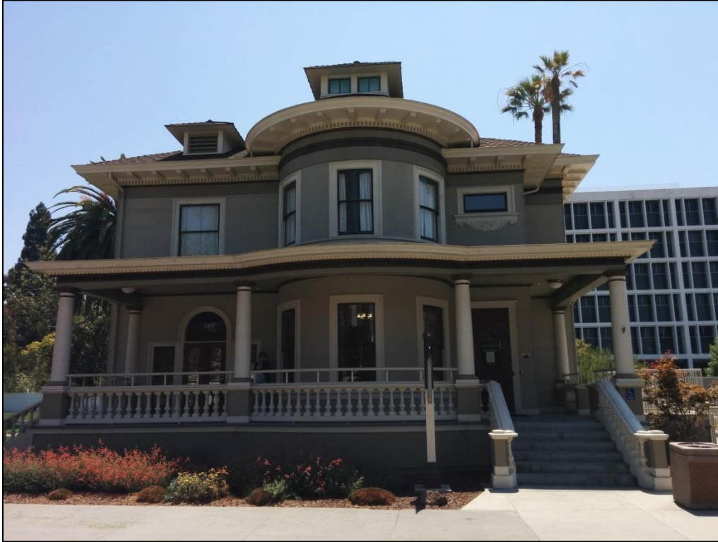
Figure 4. North-facing façade. View to the south.
