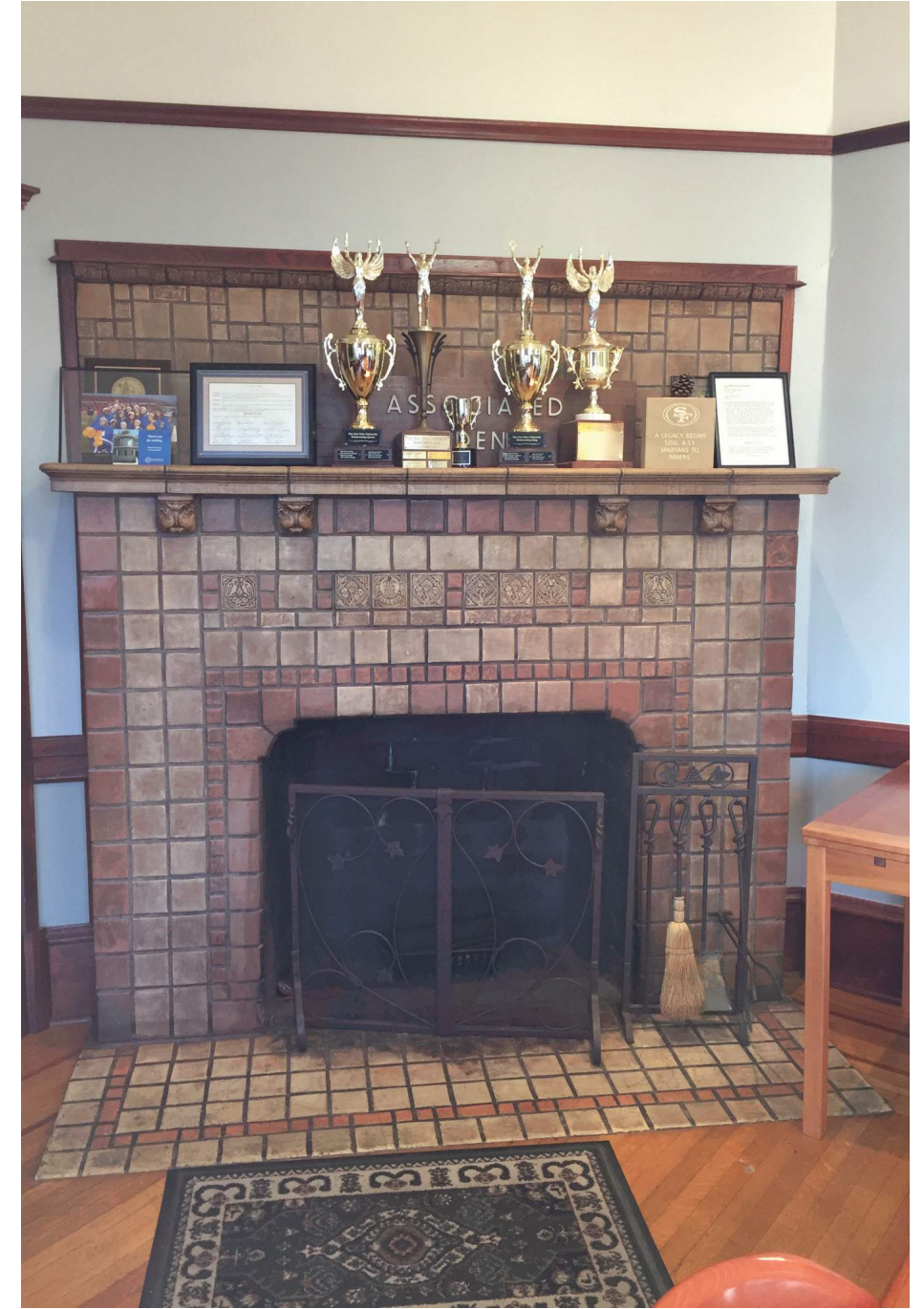
The first floor fireplace is in good condition, 2017 (Page & Turnbull)
