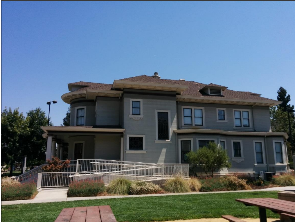
Figure 5. West elevation. View to the east.
