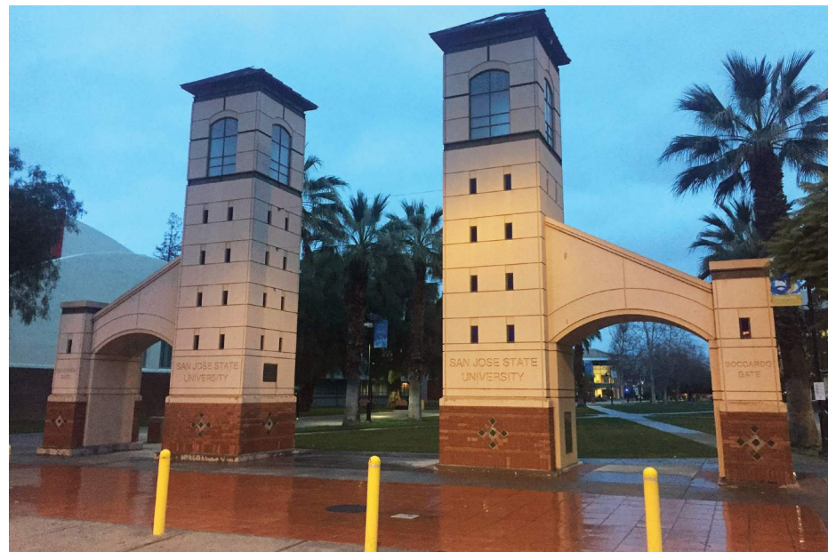
SJSU Gateway Arch at Paseo de San Carlos and S. Fourth Street, 2017 (Page & Turnbull)
