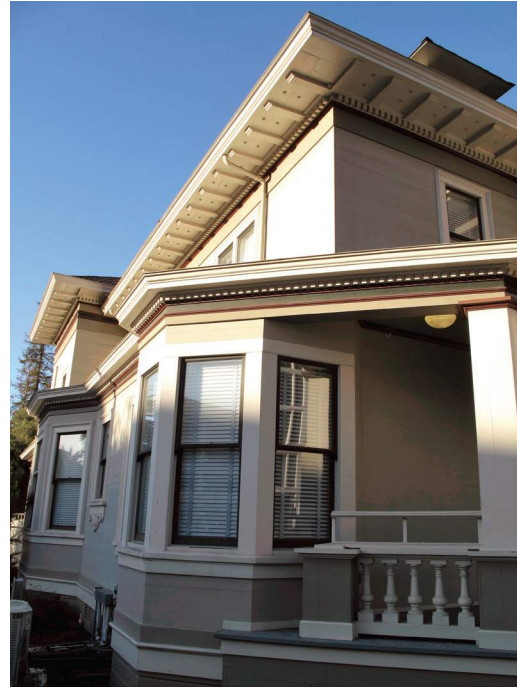
Southwest facade south side, looking northwest.
