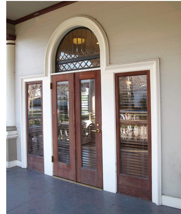
Detail of front porch door with transom and sidelites, east side.
