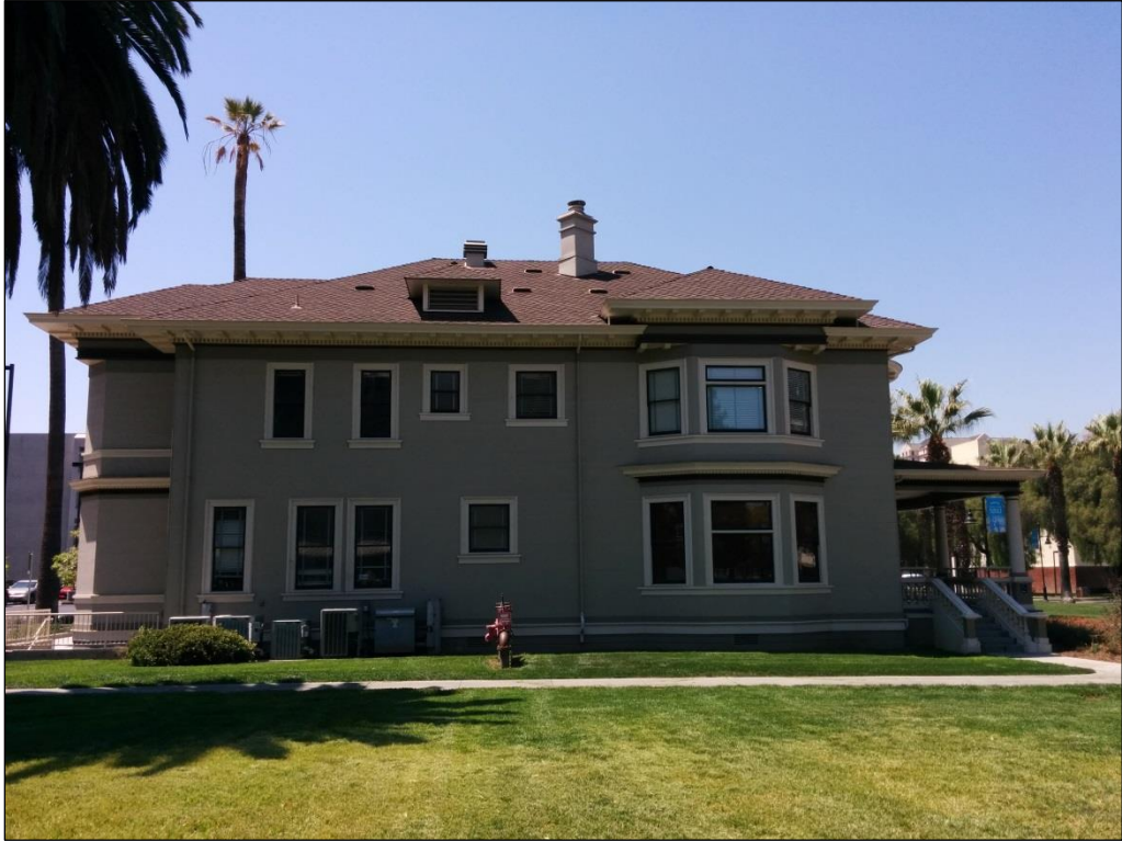
Figure 6. East elevation. View to the west.
