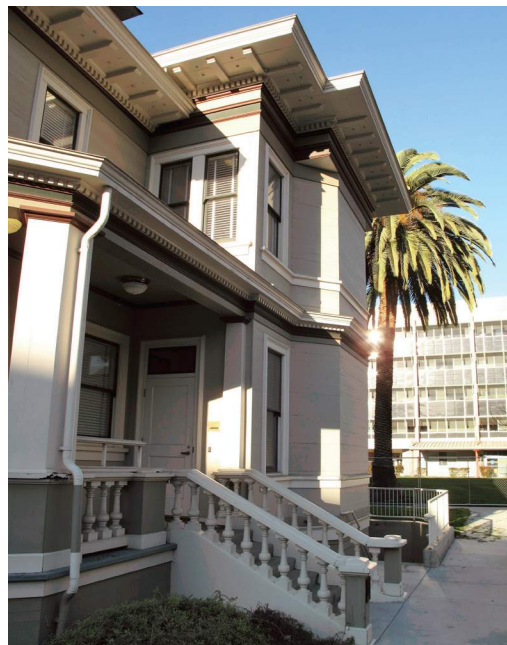
Rear (southeast) facade east side, looking northeast.
