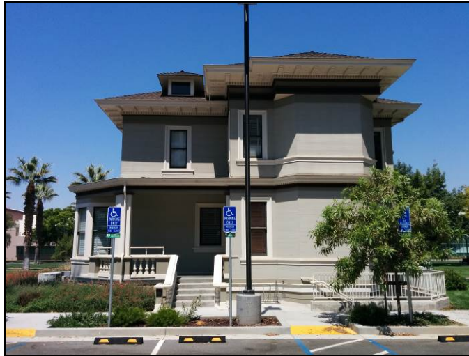
South elevation, view to the northwest
