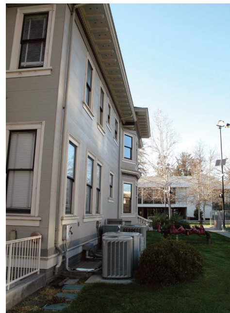
Northeast facade, looking northwest.
