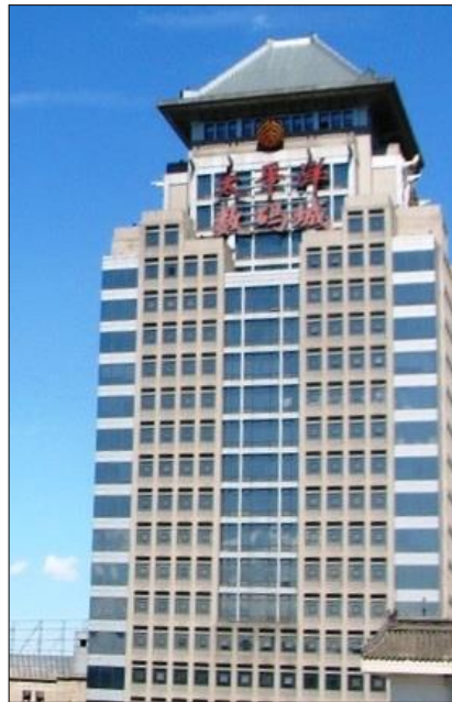
Fig. 1.11. Pacific Digital City, a “hat”-wearing building at Peking University, Beijing, China.
