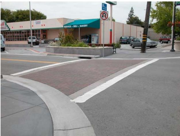
Figure 16. Example of raised sidewalk
