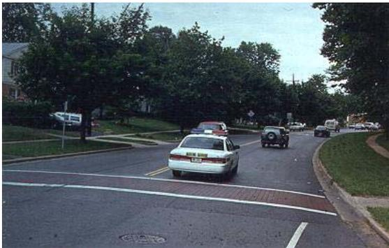
**Raised Crosswalks** are flat areas raised to the level of the sidewalk with ramps along the sides.
