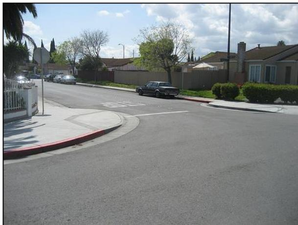
**Figure 52. Curb "bulb-out."**
