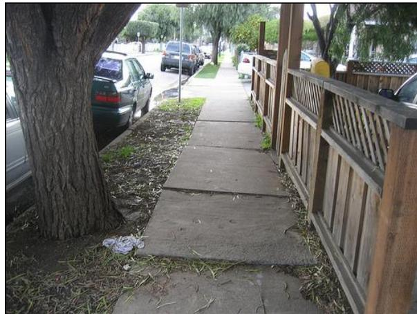
Figure 34. Sidewalk in poor condition.
