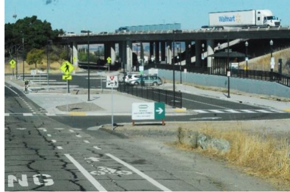
Figure 39: Current layout of Novato San Marin SMART station, facing north. Note the tight, 90-degree angle turns on the service road through the station area.
